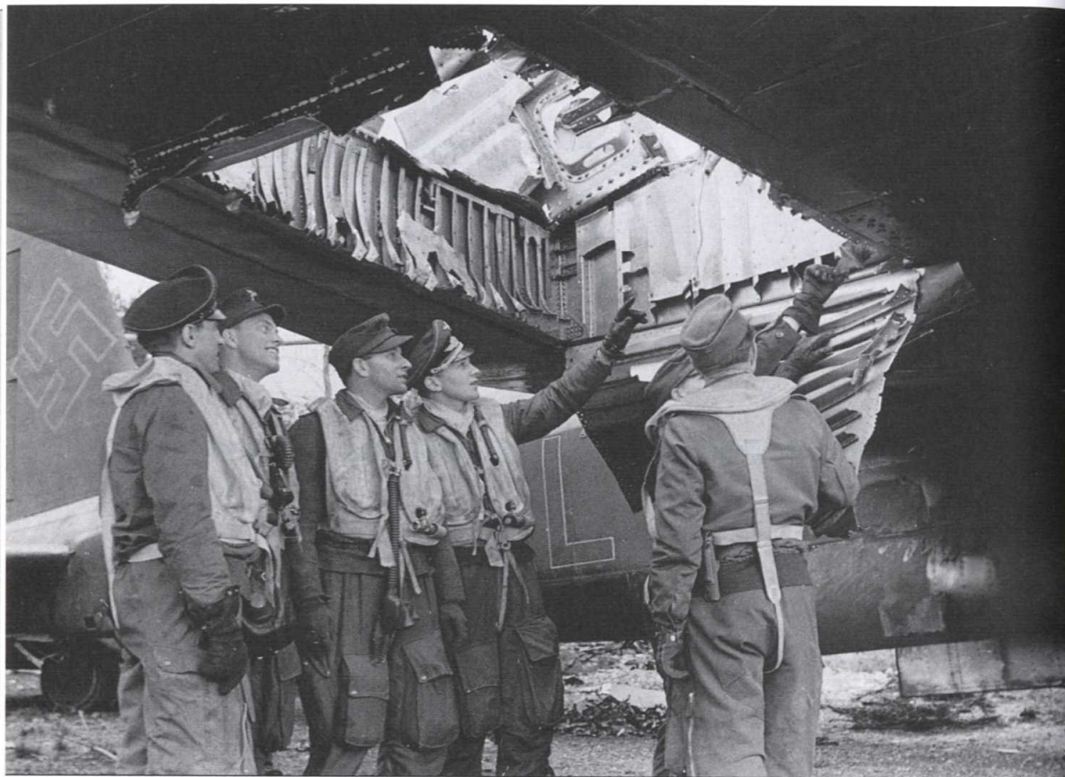
Lucky escape for crew of an He 177 crew which returned from England, after one of their bomber's fuel tanks was blown out without setting the aircraft ablaze.
