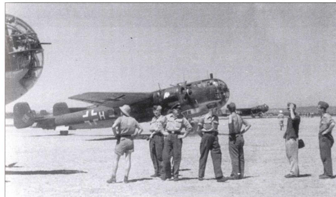
Dornier Do 217K-2s of III./KG 100. This variant, modified to carry the Fritz X, had the wing extended by just over 18 feet to provide the additional area to enable it to carry the weapon to the required release altitude. Joep
