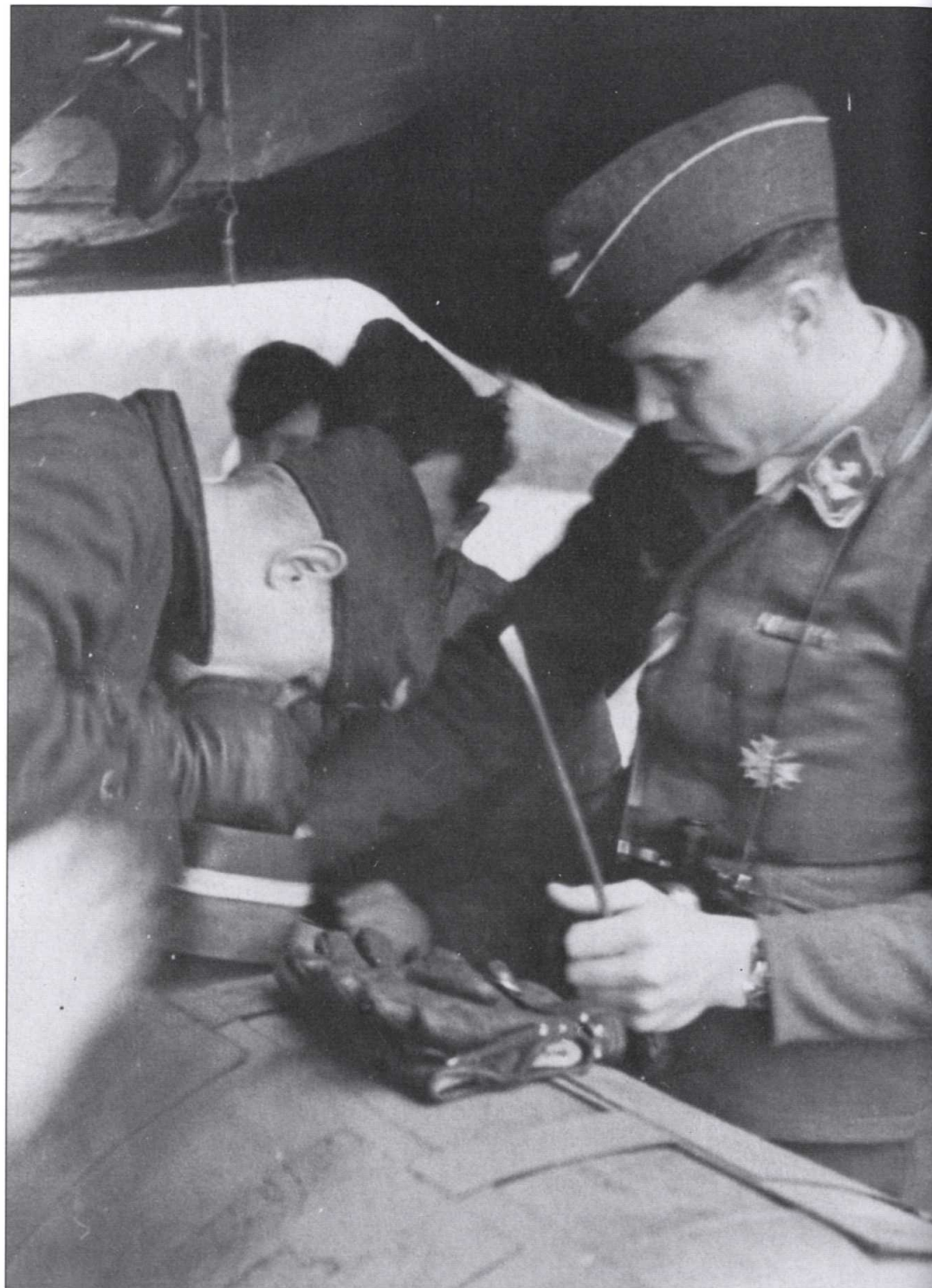
Armament NCO supervising the adjustment of the fusing system of the AB1000 incendiary bomb container.
