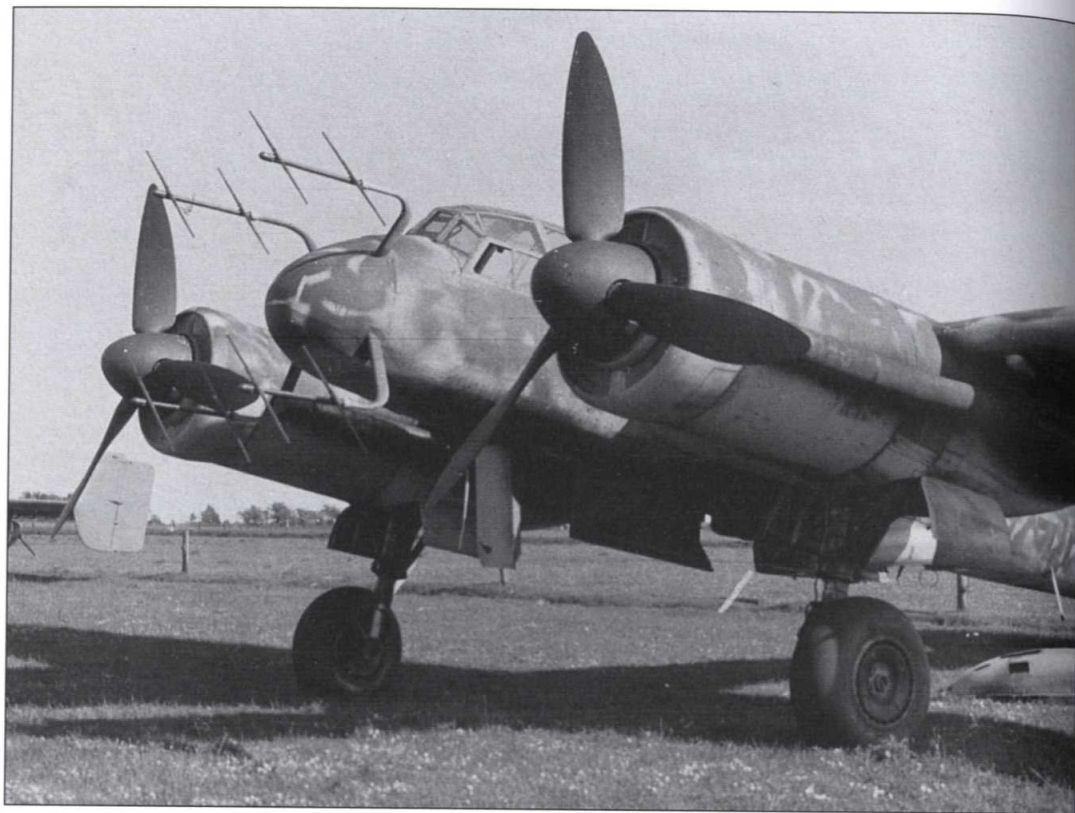
A Junkers Ju 88G fitted with SN-2 airborne interception radar.
