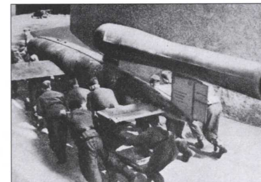
V.1 being manhandled on to the launching ramp.
