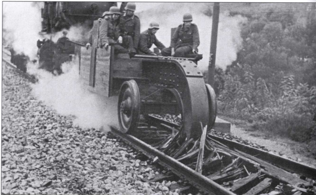
As German forces made a fighting withdrawal up the length of Italy, they carried out a systematic destruction of the infrastructure to leave as little as possible that would be of military value to the enemy. The powerful Schwellenpflug device made short work of railway tracks. via Rigelsford
