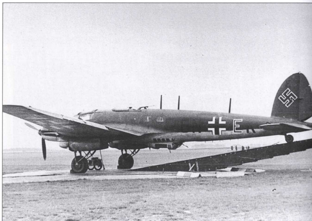
He 111s of Kampfgruppe 100 (KGr 100), the special night-attack unit which operated from Vannes in Brittany. These aircraft carried receivers for the X-Gerät beam bombing system, employing two additional aerial masts mounted on top of the rear fuselage. The system enjoyed only moderate success during attacks on Great Britain, however.
