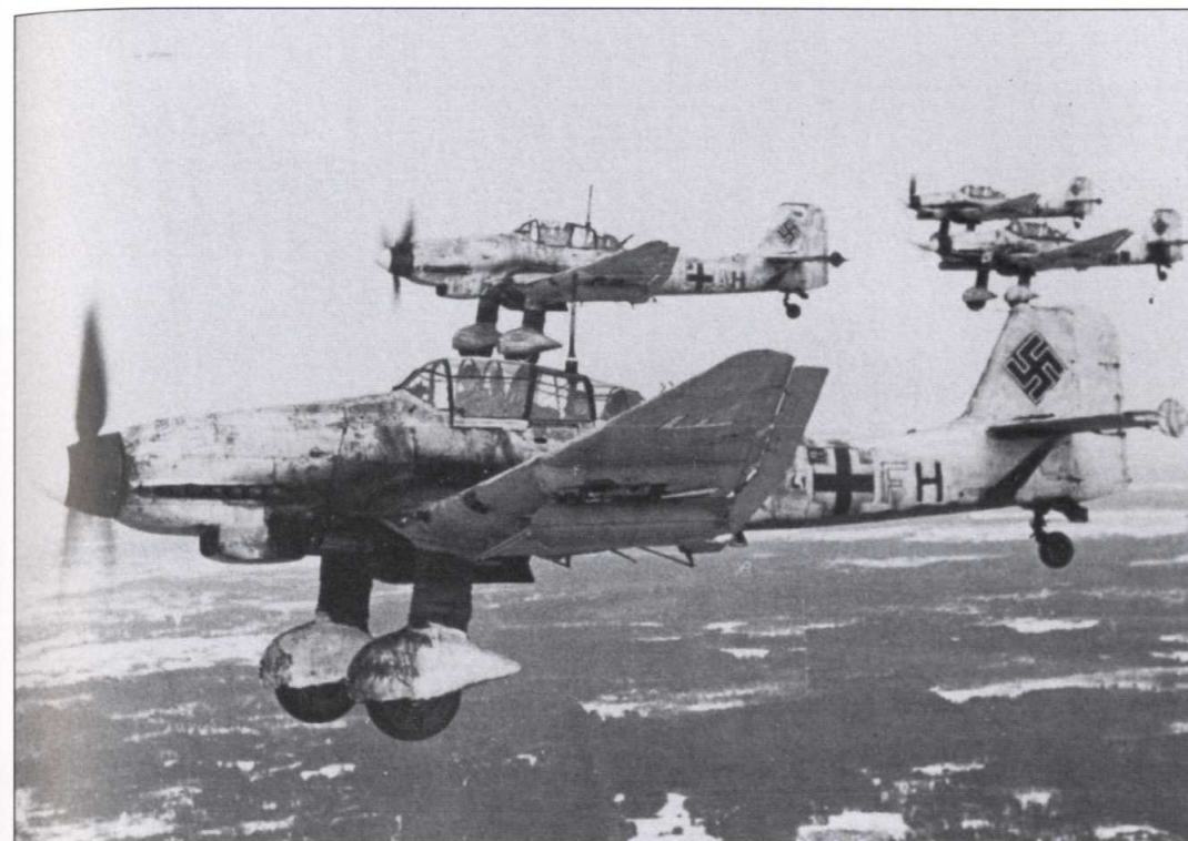
Junkers Ju 87s of 1./StG 5 on their way to a target. Each aircraft carries an AB 250 container for cluster bombs under each wing and under the fuselage. Schmidt
