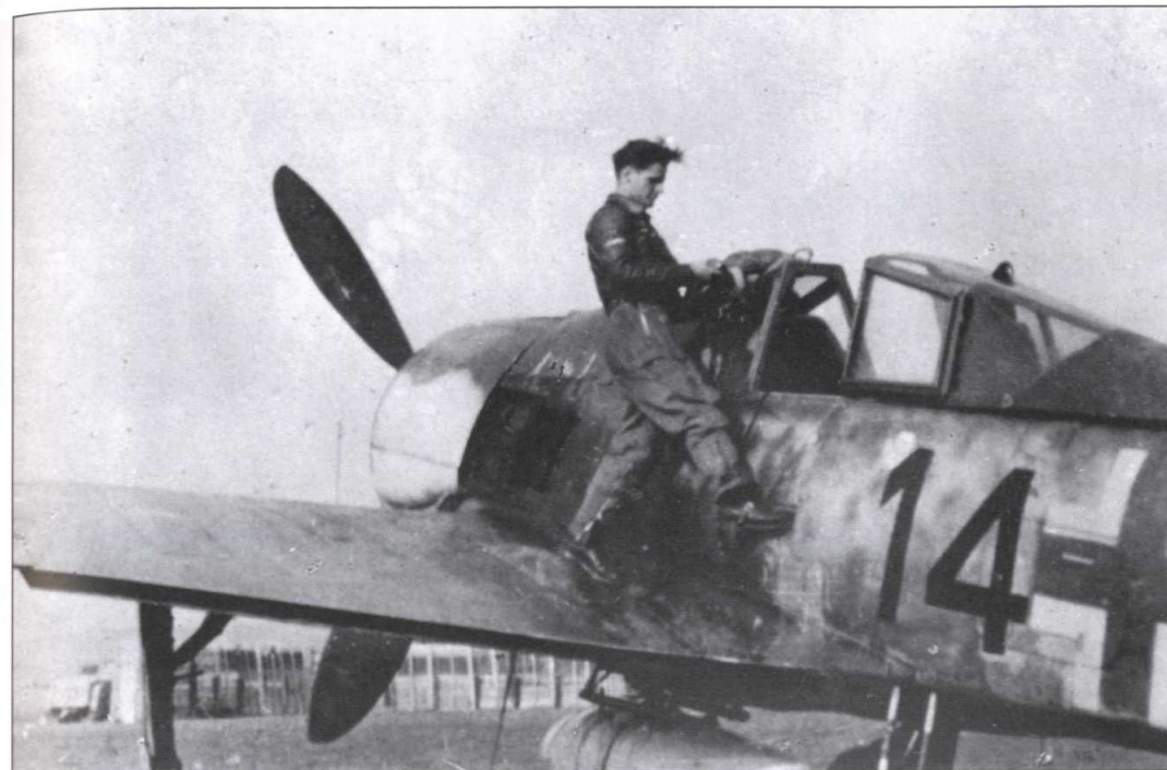
In the late spring of 1944 the Luftwaffe introduced the so-called Sturmgruppen, units operating Fw 190s fitted with additional armour and two 30-mm cannon. Flown by volunteer pilots, these aircraft were to hold tight formation and close on US heavy bomber formations from behind, braving the heavy return fire. From a range of about 100 yards they would open a withering fire on their prey. Unteroffizier Bösch of IV./(Sturm) JG 3 is seen boarding his aircraft at Schongau. Note the large slab of toughened glass fitted on the side of the canopy, indicating that this was one of the modified aircraft.
