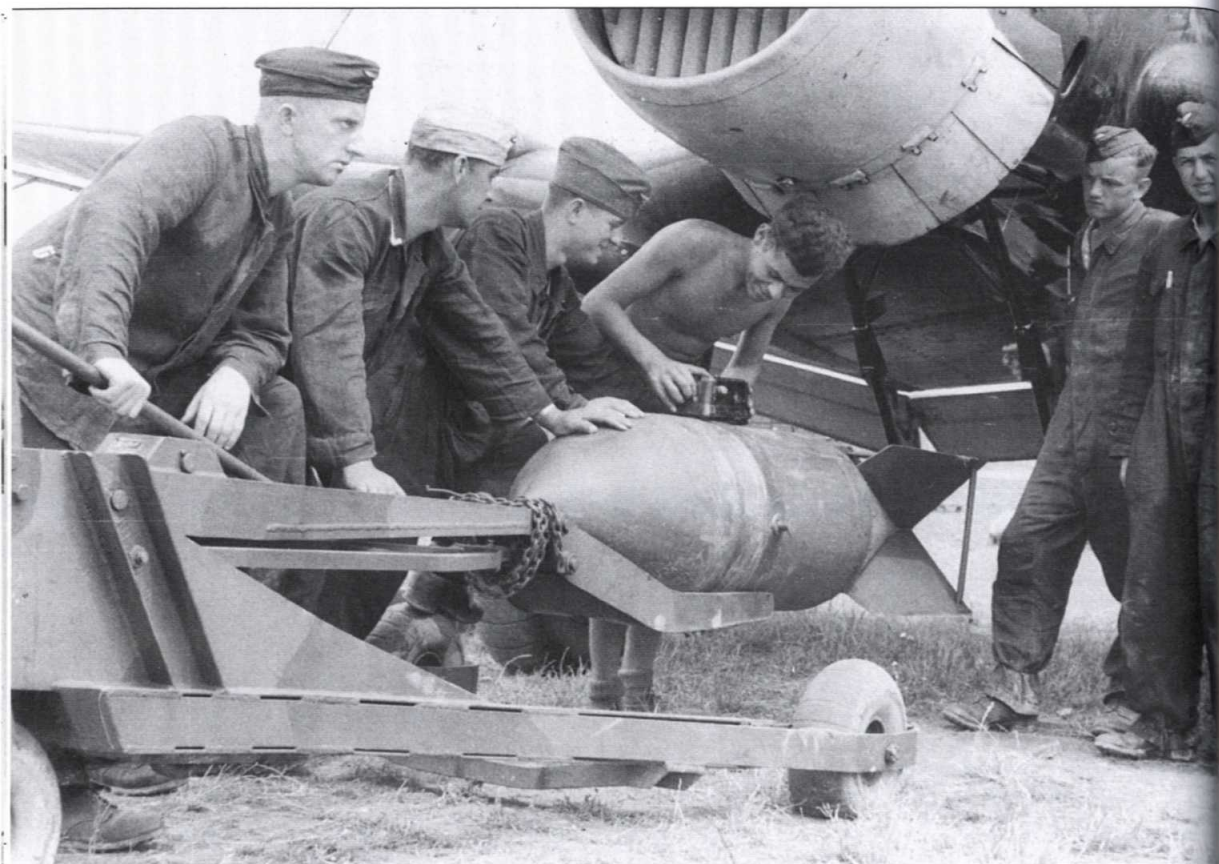
Loading an SC 250 (550-pound) bomb on the fuselage rack of a Ju 87.
